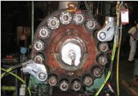
NEW METHOD: HYTORC-NUT/COLD STRETCH (16) 2-1/2" BOLTS - NEW TIME: 1 HOUR 20 MIN. OLD METHOD-PREVIOUS TIME: 8 HOURS 10 MIN. NEARLY 7 HOURS OF TIME SAVED!
