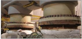
NEW METHOD: HYTORC NUT/COLD STRETCH (60) 2" BOLTS – NEW TIME: 2 HOURS 15 MIN. OLD METHOD-PREVIOUS TIME: 5 HOURS NEARLY 3 HOURS OF TIME SAVED!
