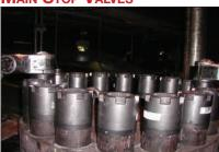
NEW METHOD: HYTORC NUT/COLD STRETCH (16) 2-3/4" BOLTS - NEW TIME: 35 MIN.
